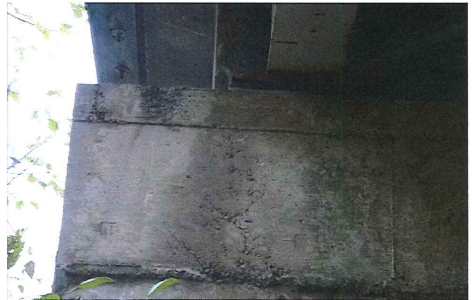
CK-2213 Woods Abutment Pier 2 Concrete
