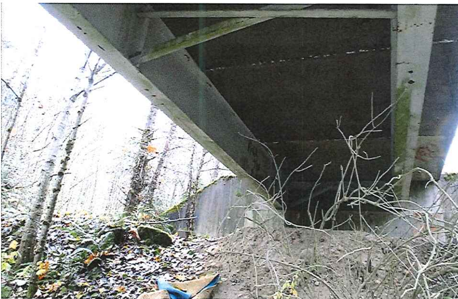
CK-2213 Span 3 and Woods Abutment
