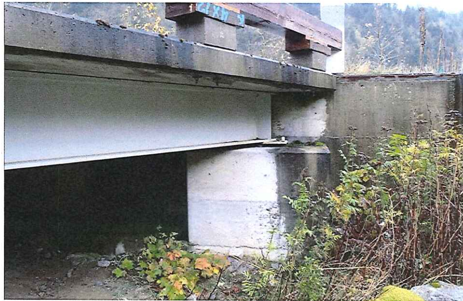
CK-2213 Camp Abutment
