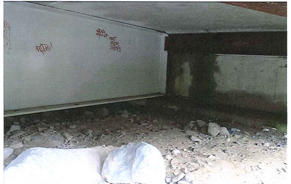
CK-2213 Camp Abutment (2)
