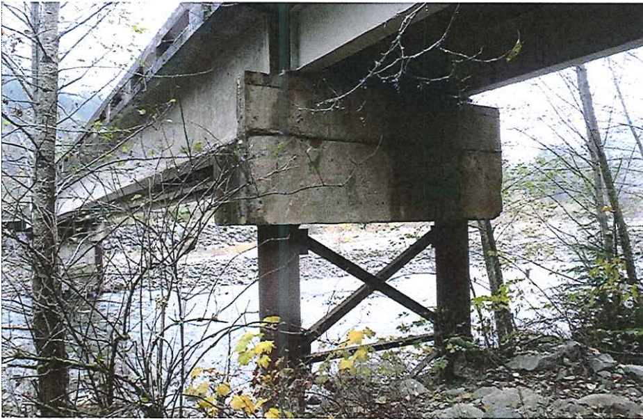
CK-2213 Span 2 and 3
